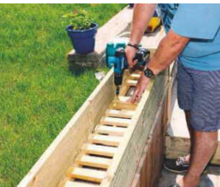
STEP 14. A series of short battens are then screwed in to the long battens
